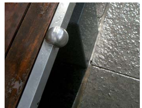
Figure 18. Studs to prevent skateboarding
